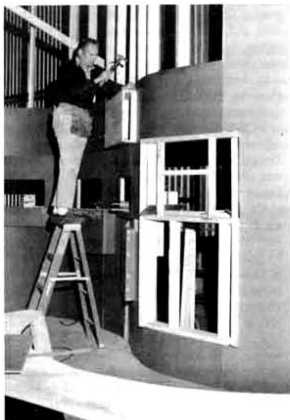
Mr. Frank L. Howard, master carpenter, works on the false walls just to the right of the hangar's visitor entrance. The framed openings will eventually contain Cunningham memorabilia.
